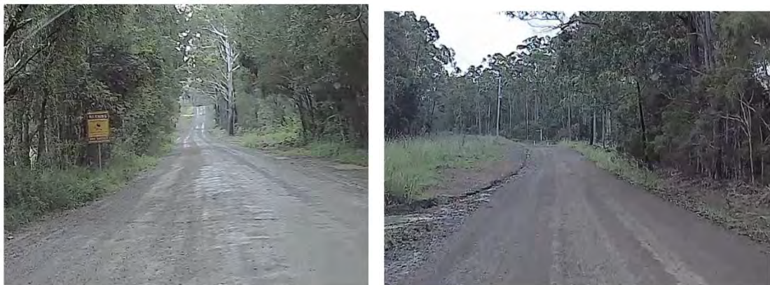
FIGURE 2.5 Typical views of Shallow Bay Road
