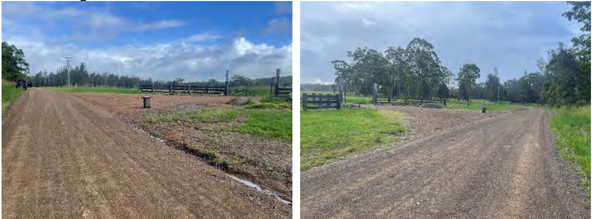
Figure 6.1 Sight distance from existing driveway looking south (L) and north (R)
