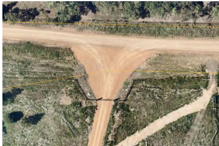
Figure 5.3 Aerial photograph of existing driveway (2023)
